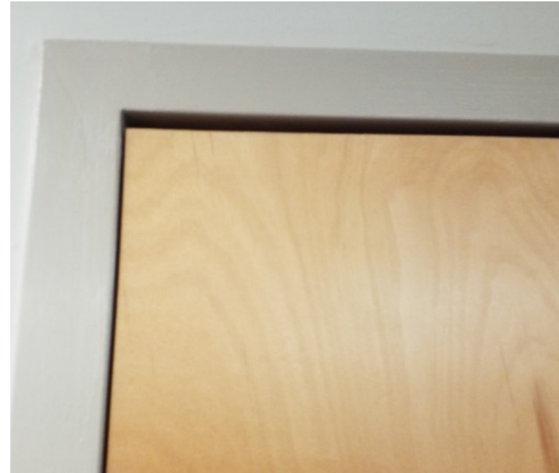
mechanical room (wood door and hollow metal frame)
