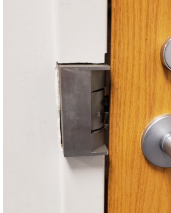
electric strike with mortise lock
