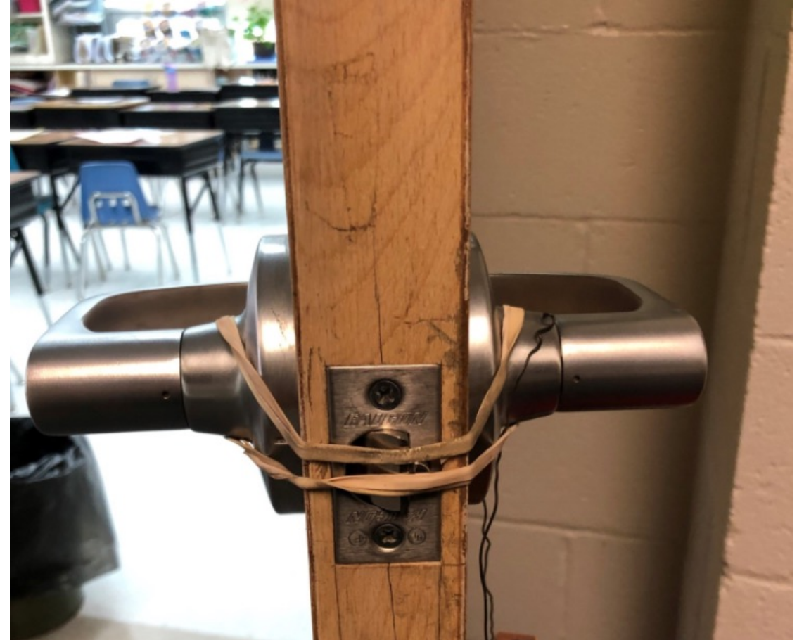
classroom wood door in hollow metal frame
